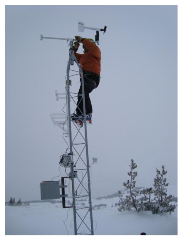
With numb fingers, Mark Staples puts up the weather station at LuLu Pass outside Cooke City. It was a frigid 2F with a 20 mph wind. It measures wind speed, direction, temperature and relative humidity. This new station was recently purchased by the **Friends of the Avalanche Center**. It sends data hourly to a web page: http://bit.ly/5yXgti
